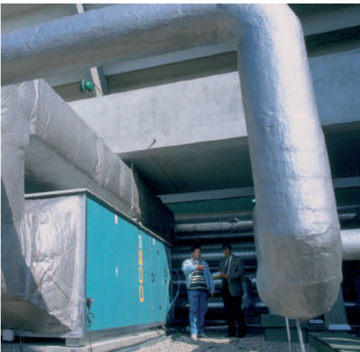
Circulating pumps for building management
