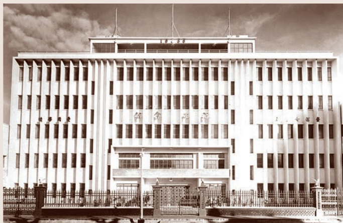
↑ Hokkien Huay Kuan Building, 1955-2001
